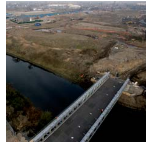
Temporary bridge on the Olympic Park
