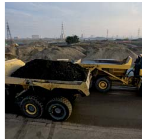
Earth being moved around the Velodrome site
