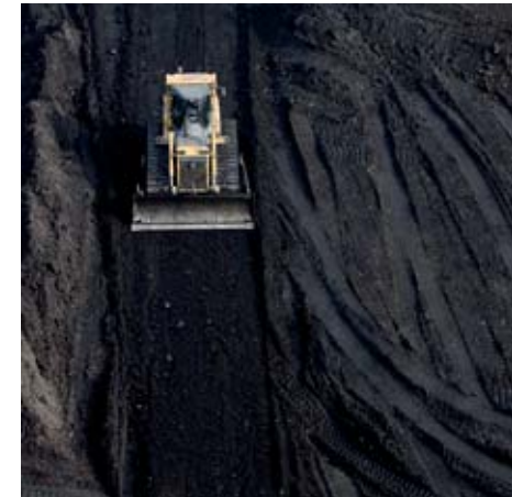
Olympic Park site being cleaned and cleared
