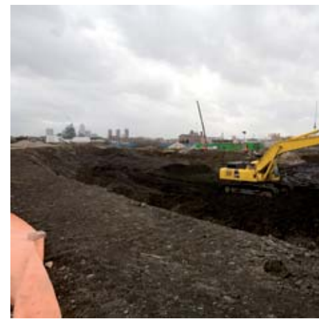
Olympic Stadium bowl being 'cut' into the ground
