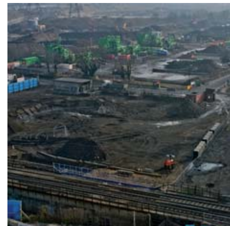
The site for the new Energy Centre
