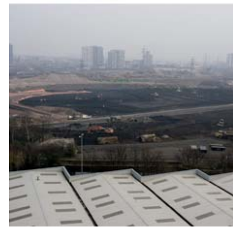
Olympic Stadium bowl takes shape
